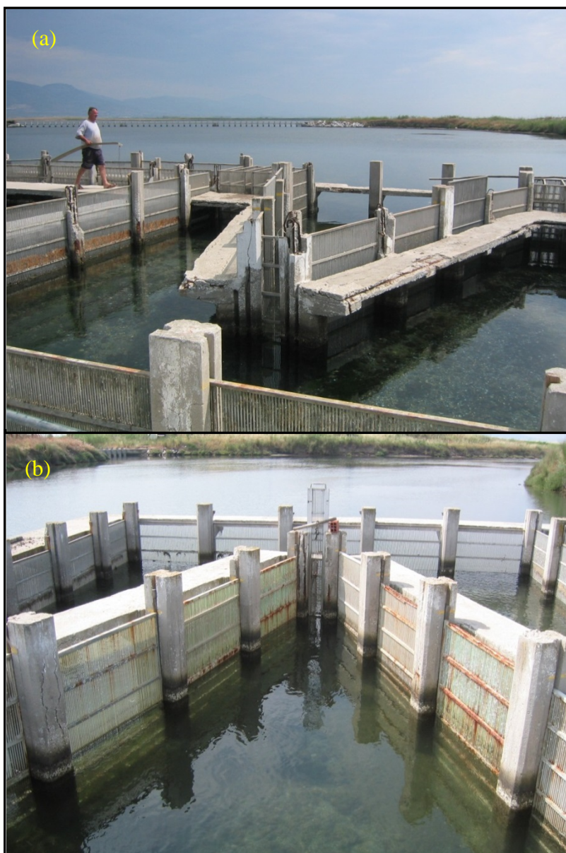
Figure 1.4.1. Modern barrier fish traps in the lagoon of Eratino (a) and in the Vassova Lagoon (b).
